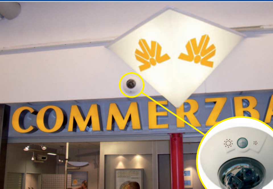
MOBOTIX D12 Dome Camera with two individually adjustable lenses.
