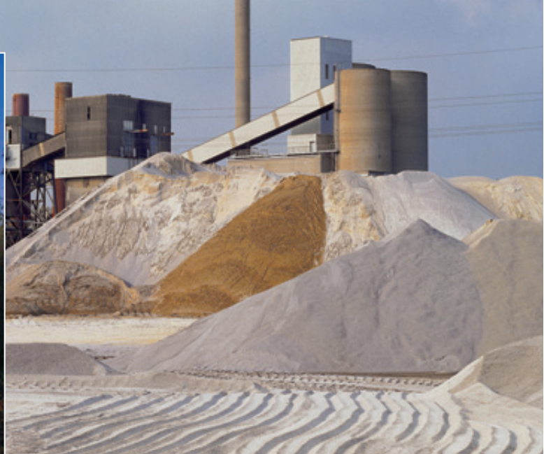
The topper kiln (left) has a daily capacity of 3000 tons.
