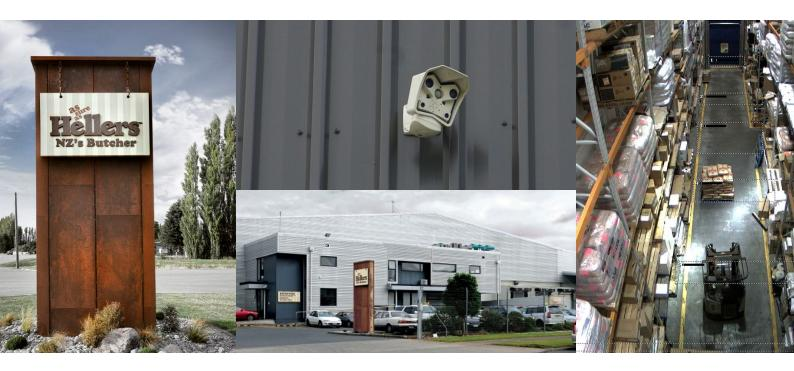
During the earthquakes and subsequent aftershocks, footage from the cameras has been used to evaluate the impact on the facility, including any damage or movement in heavy racking and large machinery. "Because the cameras are powered with PoE, a relatively small UPS was able to keep the system operation through the power outage that followed the earthquakes," Hurford mentioned "this allowed uninterrupted coverage of the factory and assisted in the engineering assessment of the facility."
