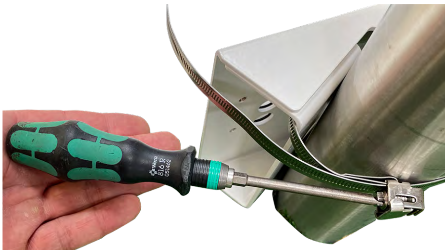
Fig. 44: Tighten the straps
