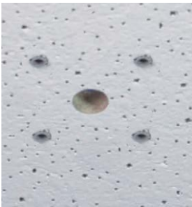
Fig. 16: Holes ready for mounting
