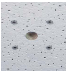
Fig. 14: Holes ready for mounting
