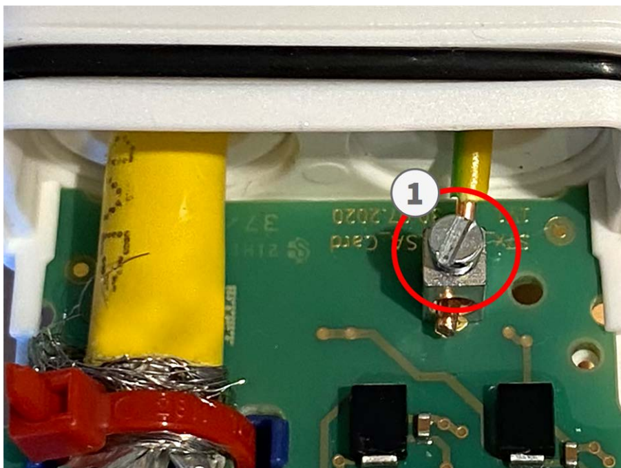
Fig. 29: Ground wire connected to terminal
