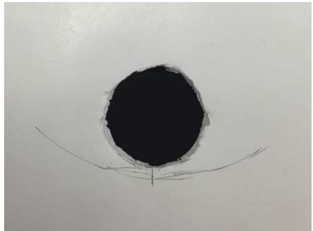
5. Drill a hole slightly smaller than the supplied plastic dowel on each marked screw hole. Then insert the plastic dowels into the drilled holes.
