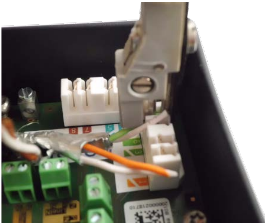
Fig. 63: Network wires connected using LSA+/Krone tool
