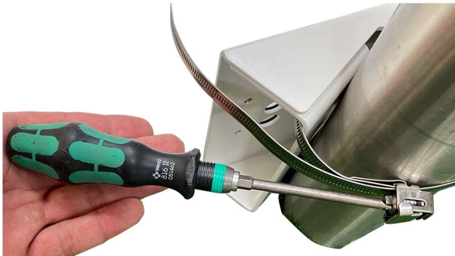
Fig. 42: Tighten the straps
