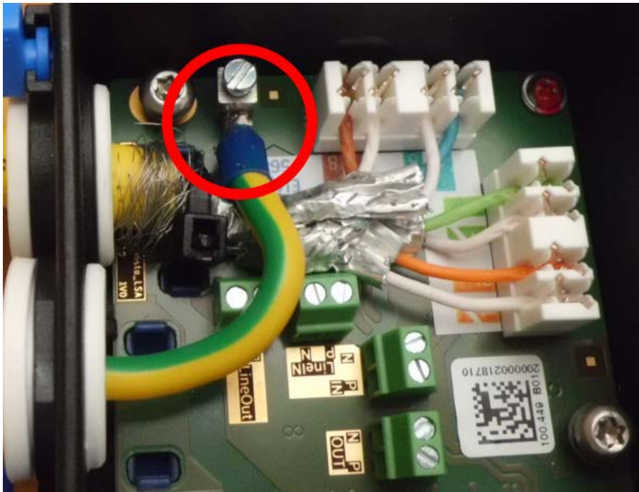
Fig. 66: Ground wire connected to terminal
