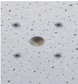
Fig. 16: Holes ready for mounting
