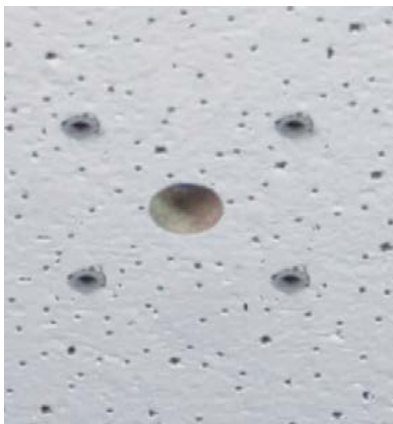
Fig. 14: Holes ready for mounting
