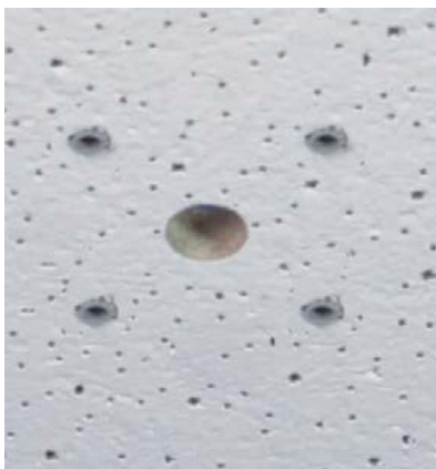
Fig. 16: Holes ready for mounting
