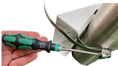
Fig. 14: Tighten the straps
