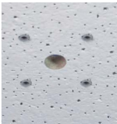
Fig. 13: Holes ready for mounting
