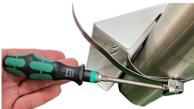
Fig. 14: Tighten the straps
