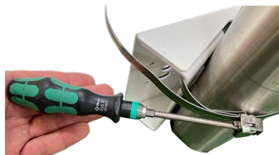
Fig. 14: Tighten the straps
