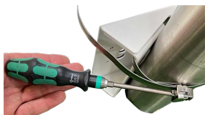
Fig. 14: Tighten the straps
