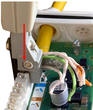
Fig. 13: Network wires connected using LSA+/Krone tool
