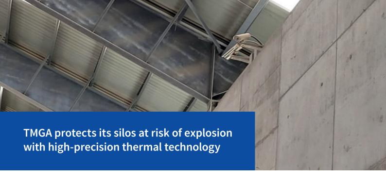
In the face of latent risks such as spontaneous combustion or explosive dust, highly sensitive thermal sensors and the Thermal Validation App provide preventive protection for the critical facilities of Terminales Marítimos de Galicia (TMGA), optimizing costs and complying with the strictest industrial safety requirements.
