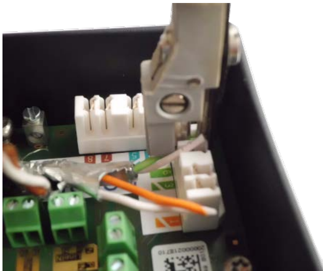
Fig. 27: Network wires connected using LSA+/Krone tool
