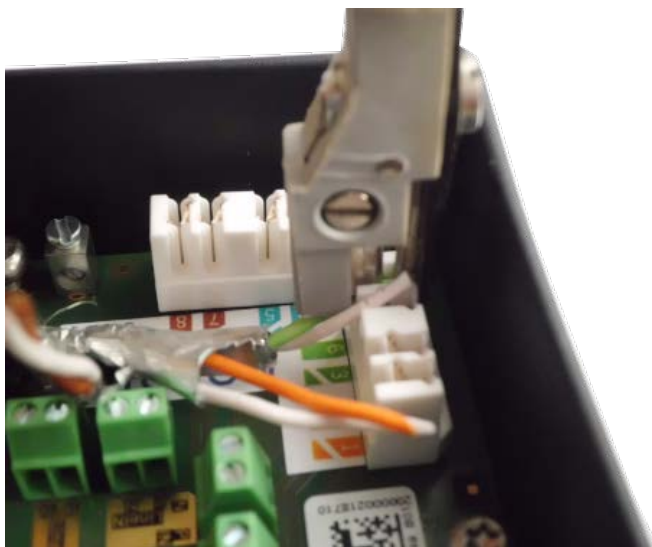
Fig. 27: Network wires connected using LSA+/Krone tool
